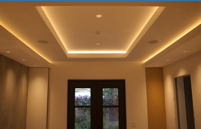
Cove Lighting using LinR12-ST-27k
